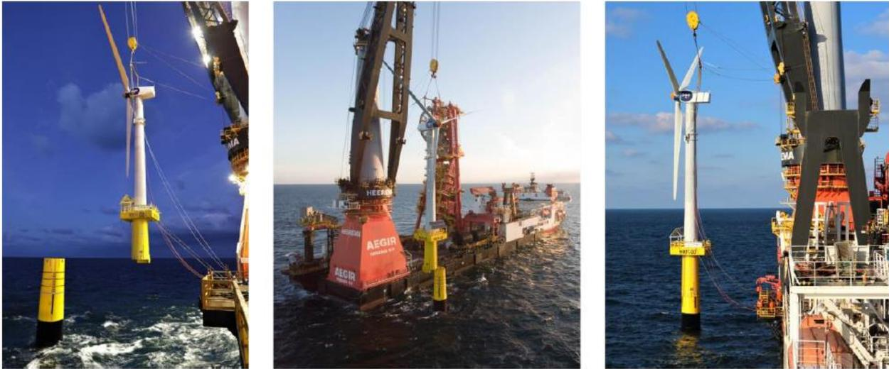
FIGURE 5 | INSTALLATION OF SLIP JOINT IN PROGRESS
